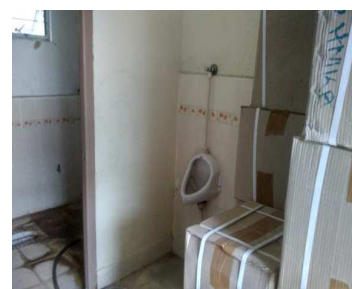
Stock of drugs and medicines being accommodated in toilet at CMS, Warangal
